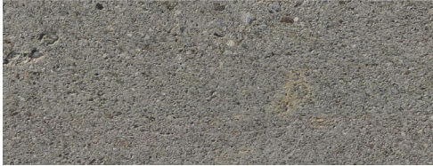
Balcony without waterproofing membrane
