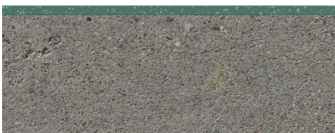
Balcony with liquid plastic or bituminous waterproofing membrane
