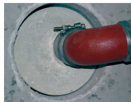
Connecting the SML pipe
