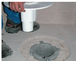
Applying the WAL-SELECTA floor drain
