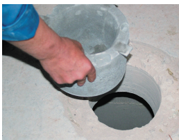
Inserting the ACO FIT-IN installation kit
